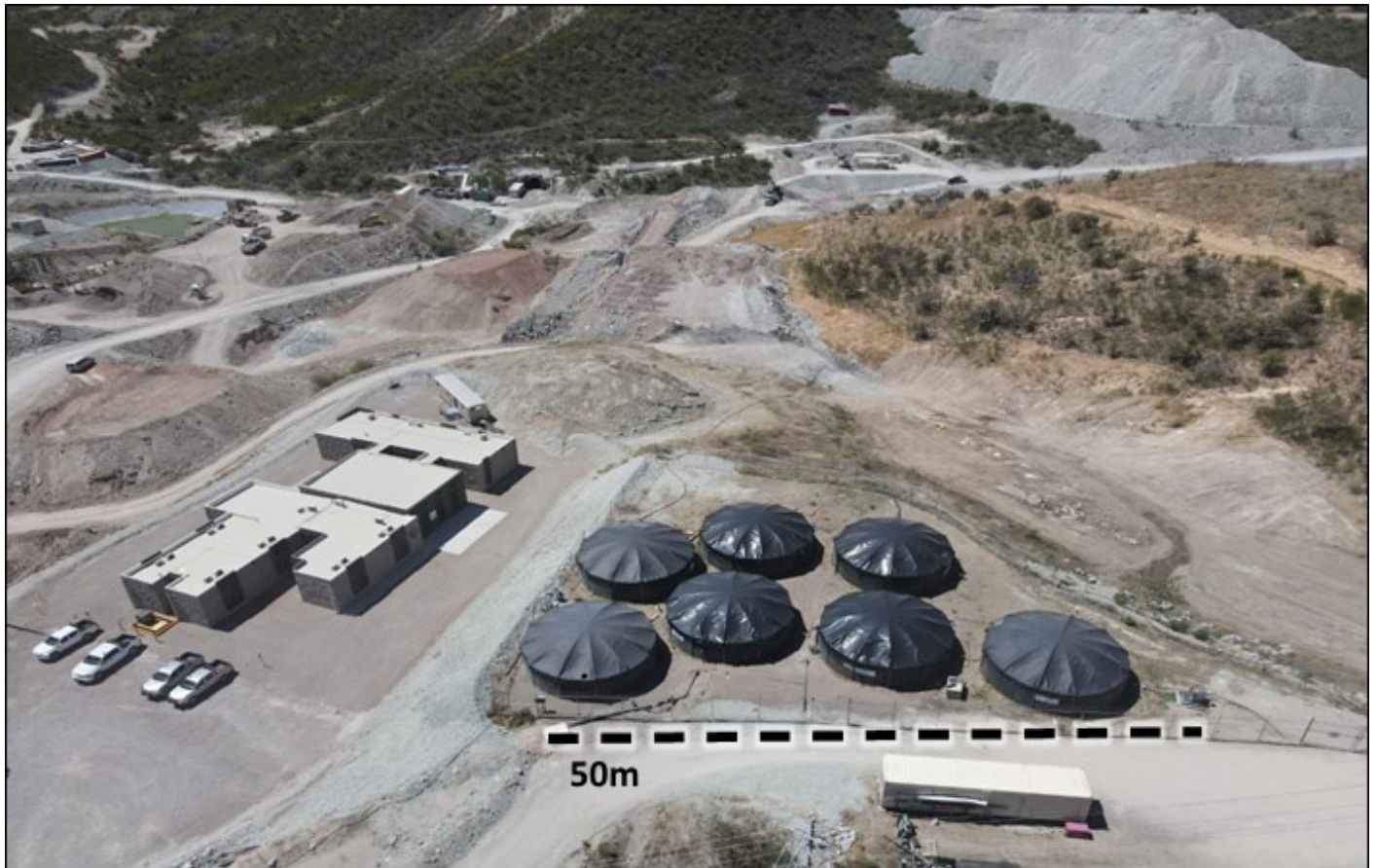
Figure 4-2: Water Distribution Tank Located Near the Main Office
