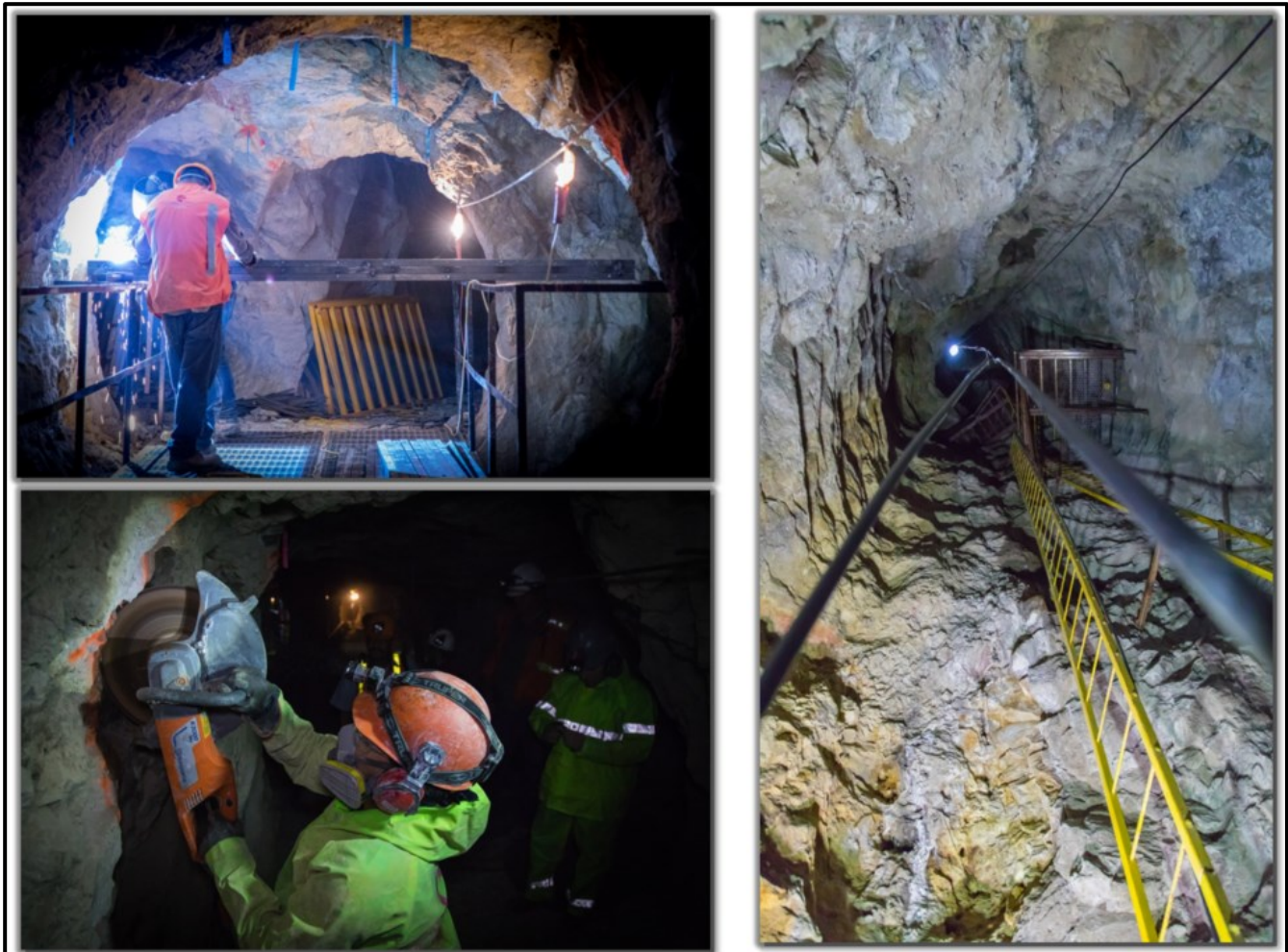
Figure 7-1: Photos of Las Chispas Underground Rehabilitation Activities
