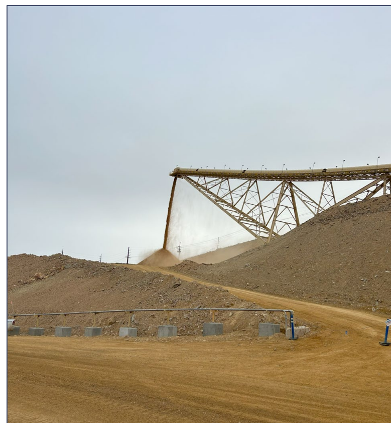
First rock through the secondary crusher
