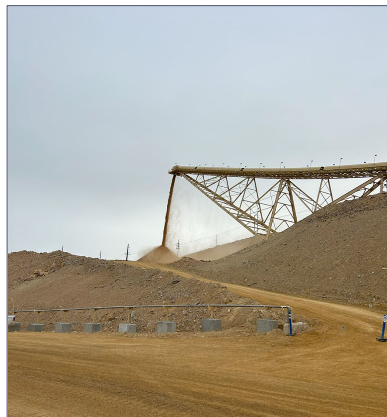
First rock through the secondary crusher
