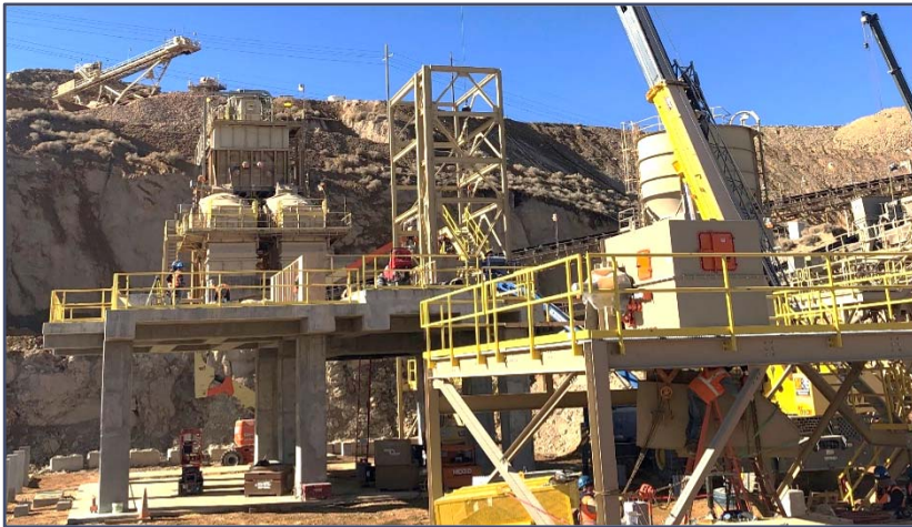
Initial high pressure grinding roll ("HPGR") installation
