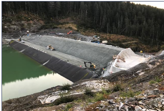
Stage 3 Dam Raise Construction
