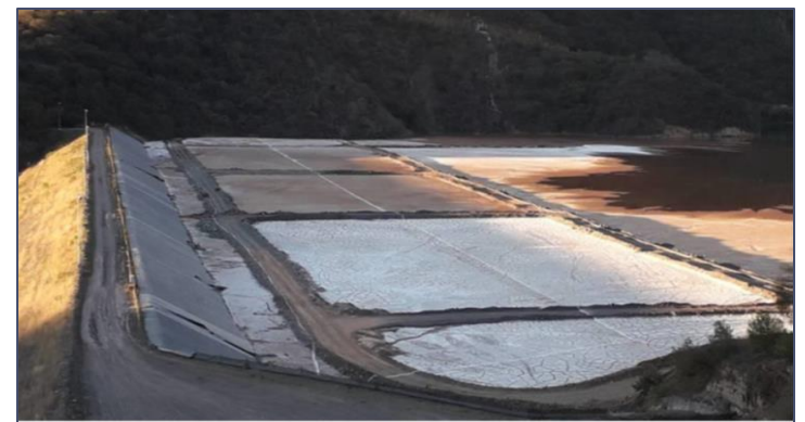
Preparation for Modified Centerline Construction Dam Raise
