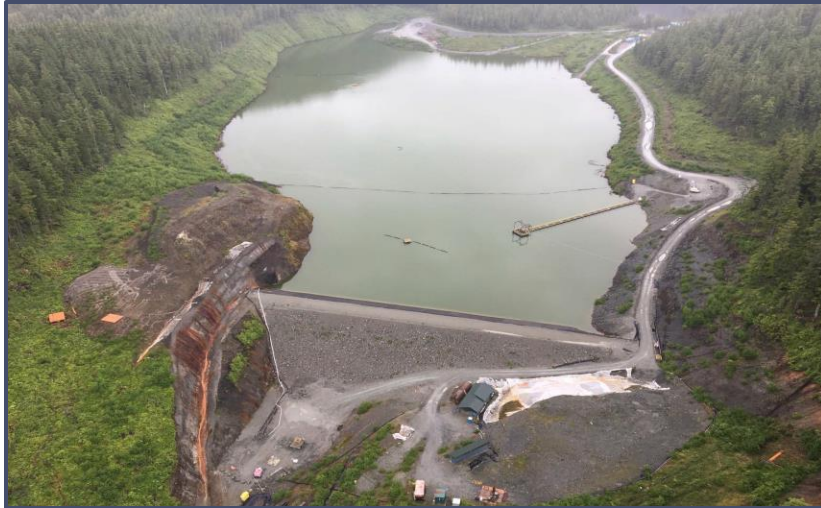
TTF – Pre Stage 3 Construction (2017)
