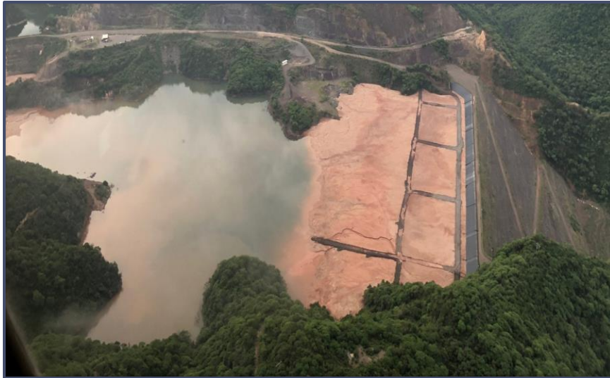
Downstream Construction & Strong Beach Formation
