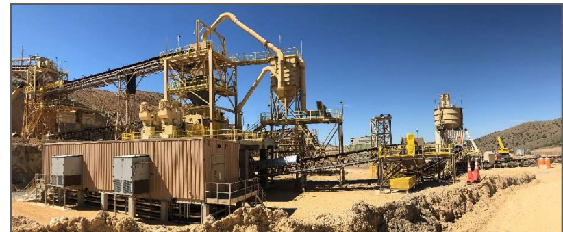
HPGR crushing unit at Rochester
