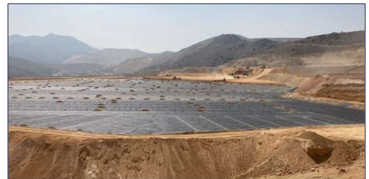
Recently constructed inter-lift liner
