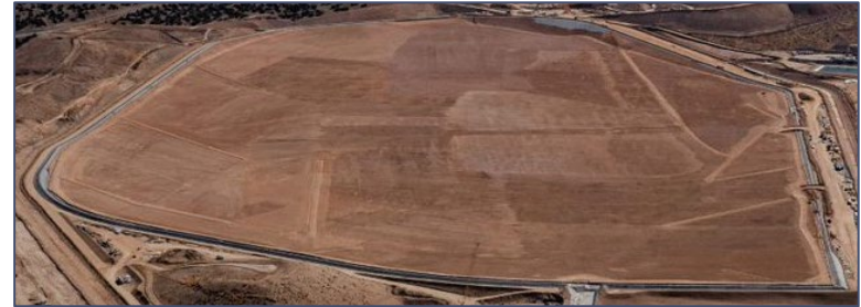
Completed Heap Leach Pad VI
