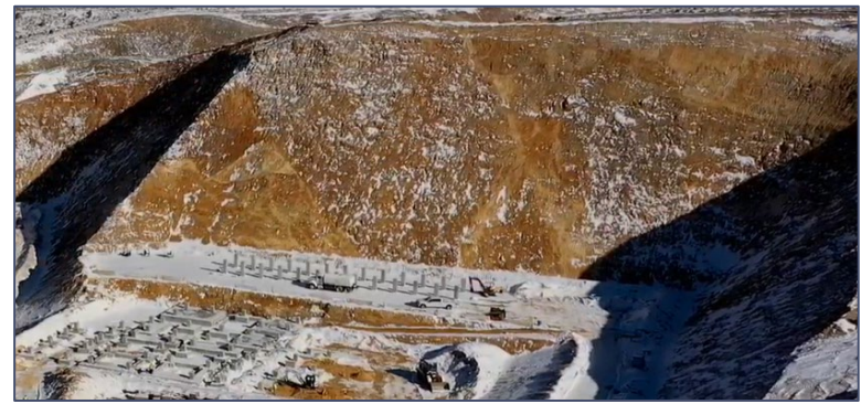
Completed Pre-screen Excavation with Foundations Well Underway
