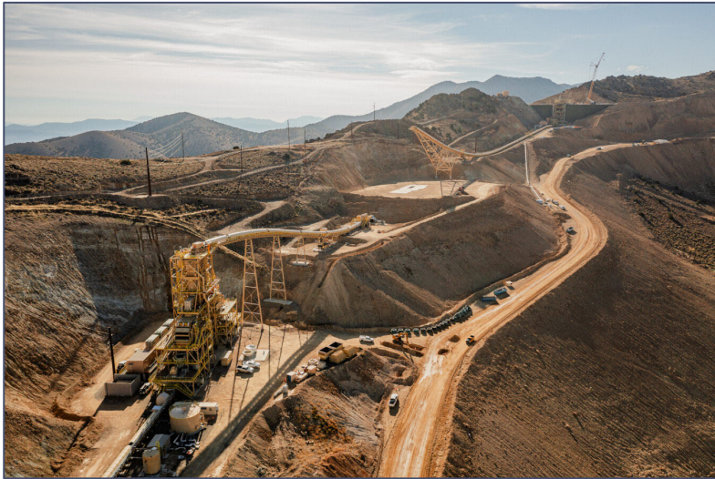
Primary and Secondary Crusher
