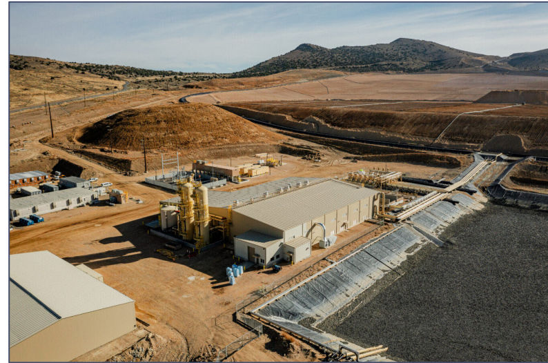
Merrill-Crowe Process Plant
