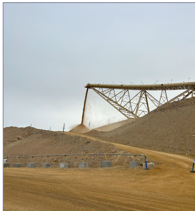
First rock through the secondary crusher
