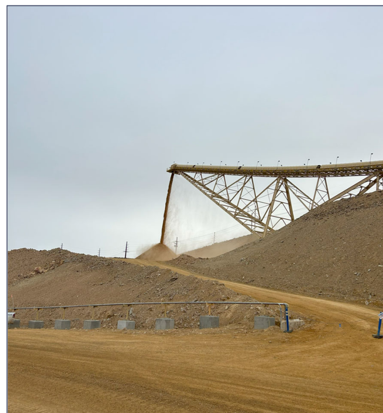
First rock through the secondary crusher
