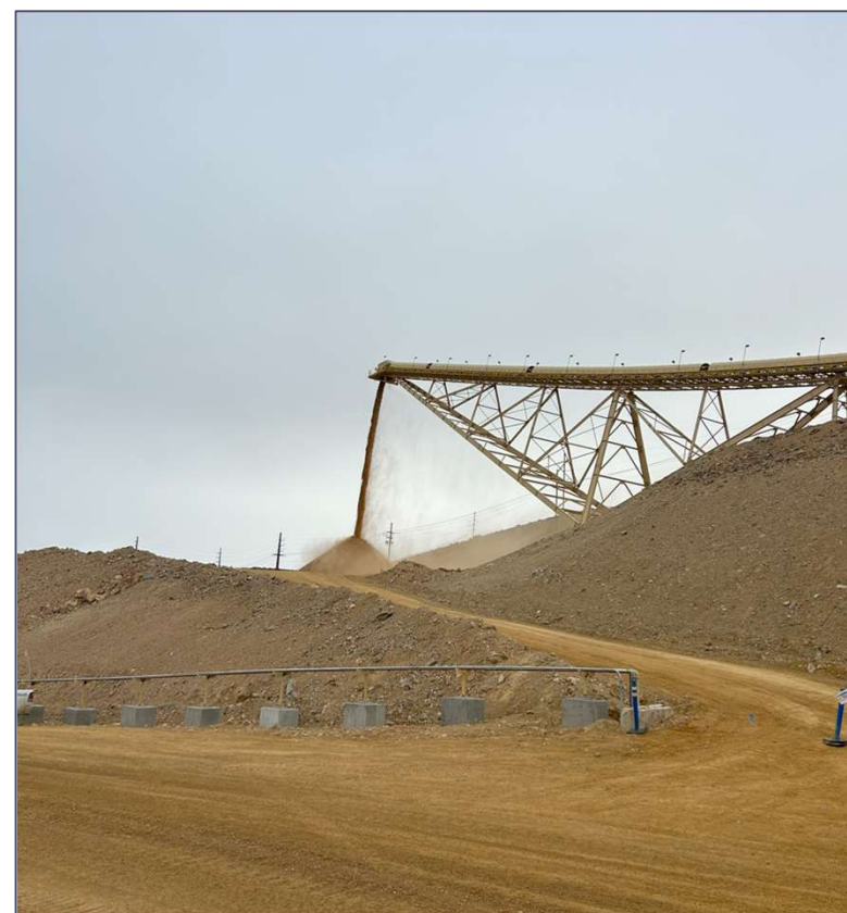
First rock through the secondary crusher
