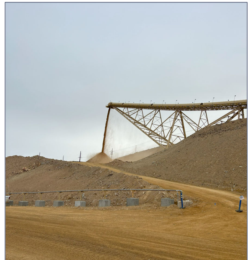
First rock through the secondary crusher
