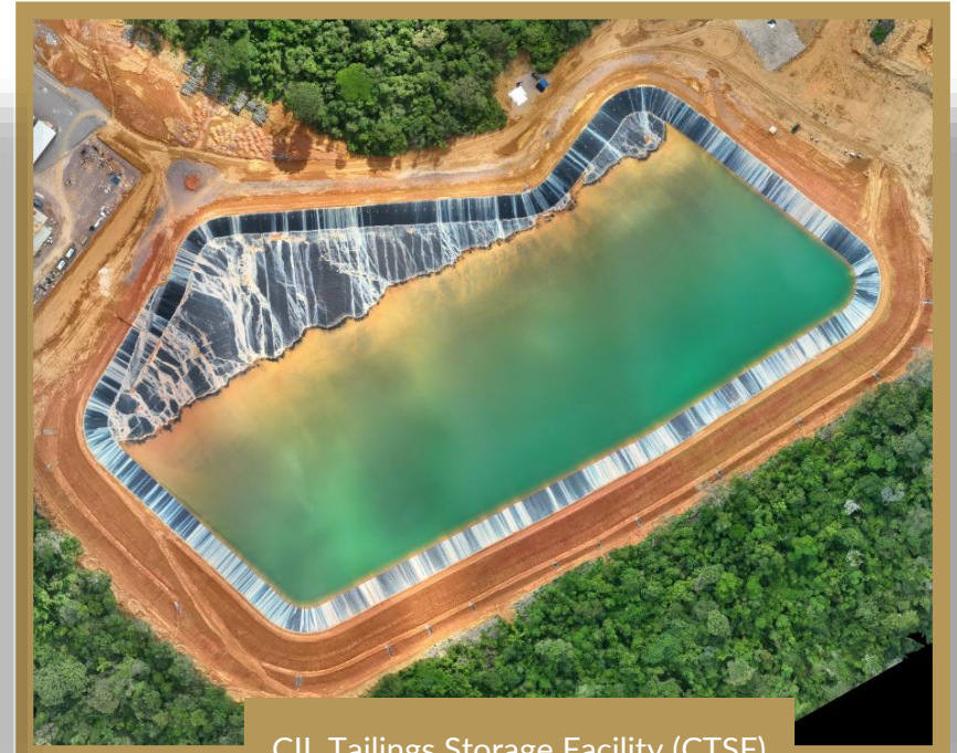
CIL Tailings Storage Facility (CTSF)
