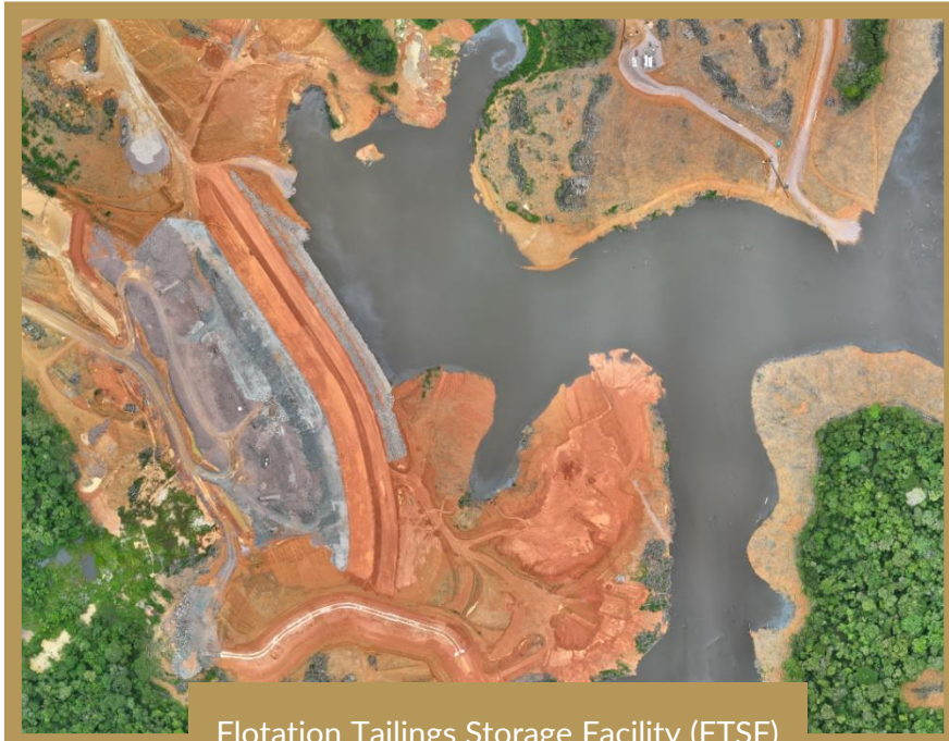
Flotation Tailings Storage Facility (FTSF)
