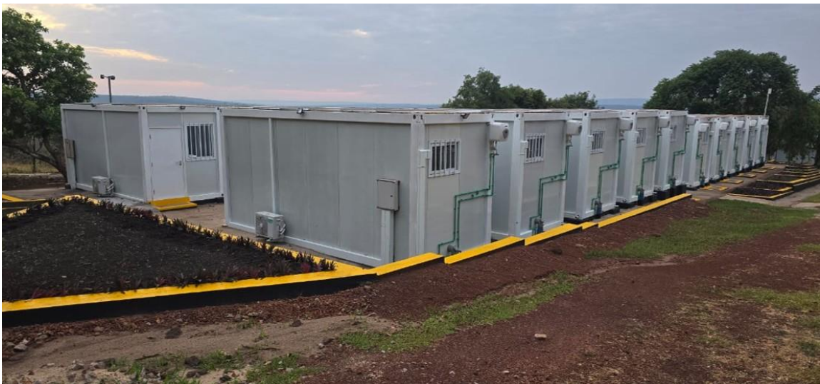
Figure 5: Kabanga camp prefabricated accommodation units
