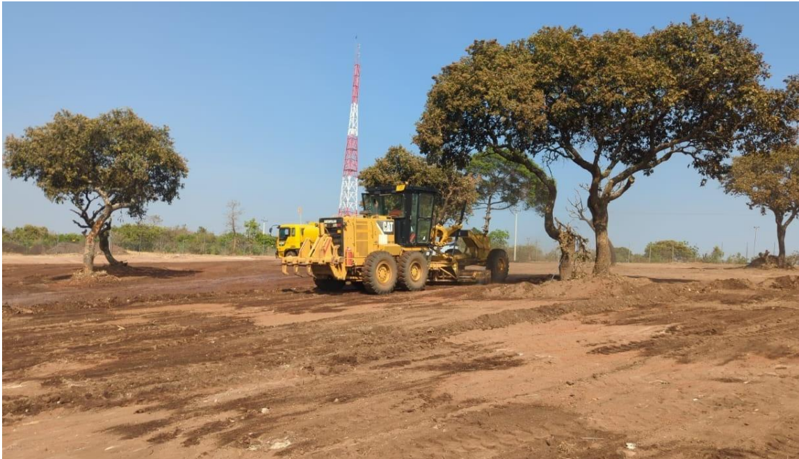
Figure 4: Laydown area grading and compaction for leveling
