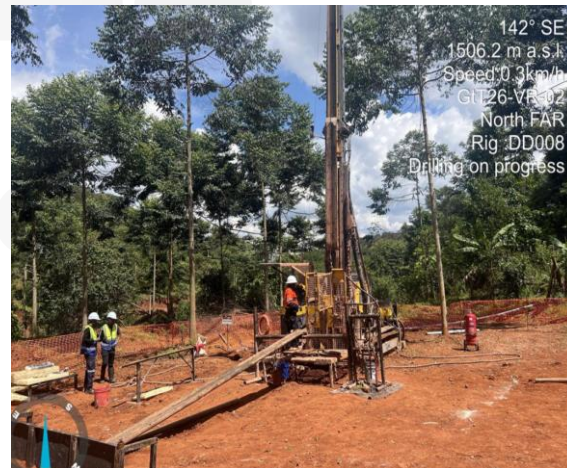
North vent raises, geotechnical hole at the North box cut
