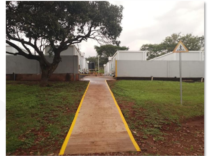
Accommodation renovations at Kabanga including painting, water and power connection
