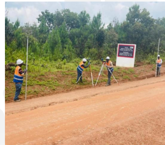
AGS conducting levelling on Project Area access road at Mpigi
