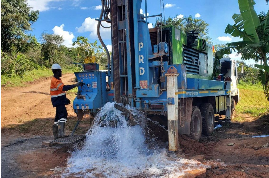
Figure 4: Production water borehole drilling at Kabanga Site, 132m deep, providing a yield of 28,000 L/H
