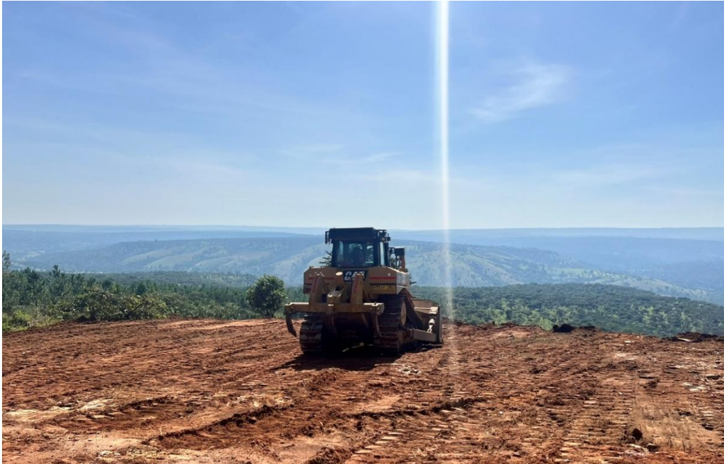
Figure 3: Project area land clearing
