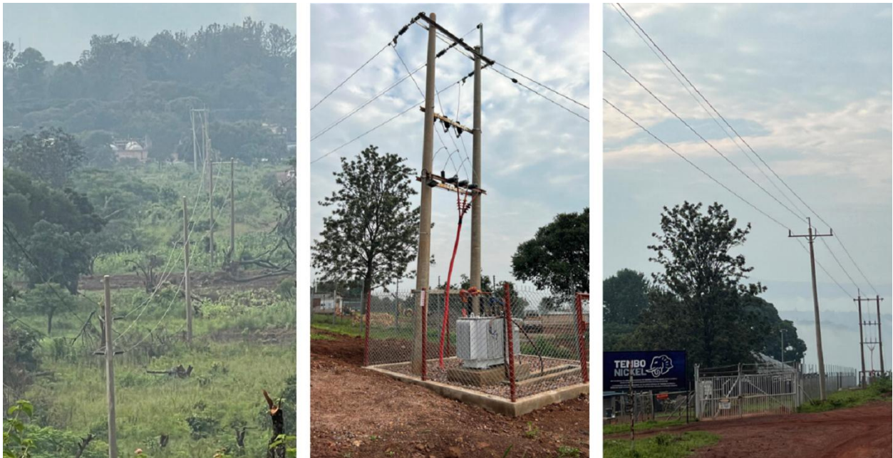
Figure 5: Images of the 33-kilovolt power line connecting the Kabanga camp to the regional power grid.
