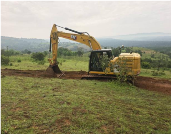
Access road preparation to test pit 05 at the north box cut waste rock dump
