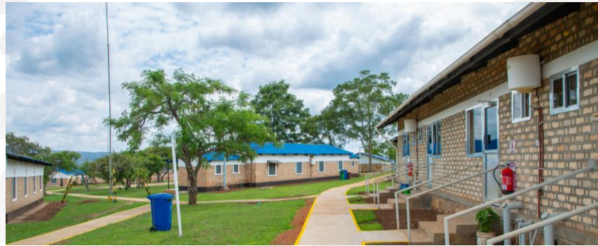
Accommodation renovations at Kabanga
