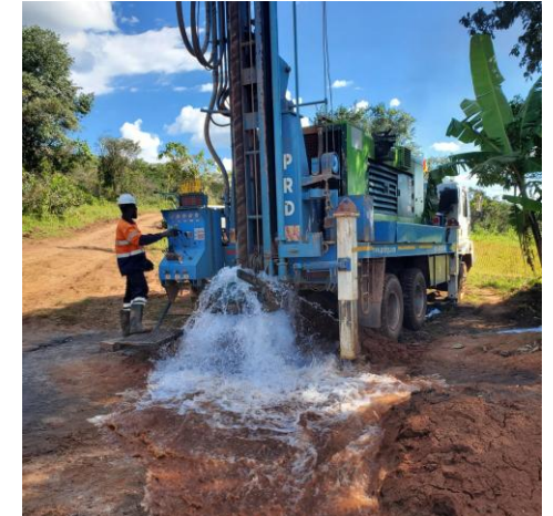
Production water borehole drilling at Kabanga Site, 132m deep, providing a yield of 28,000 L/H
