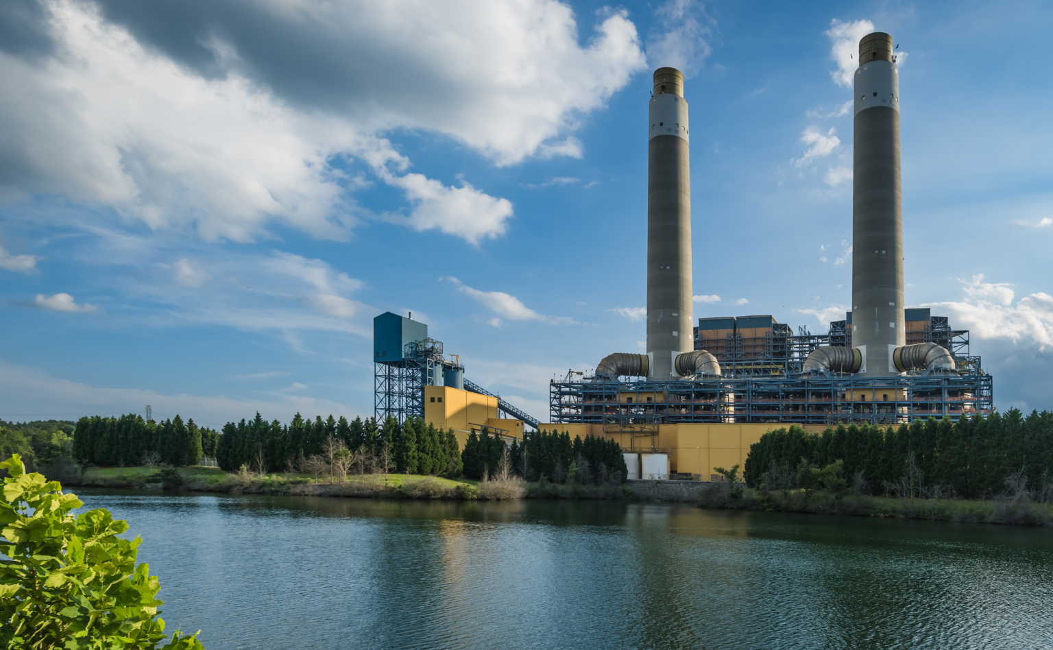
Belews Creek Steam Station
