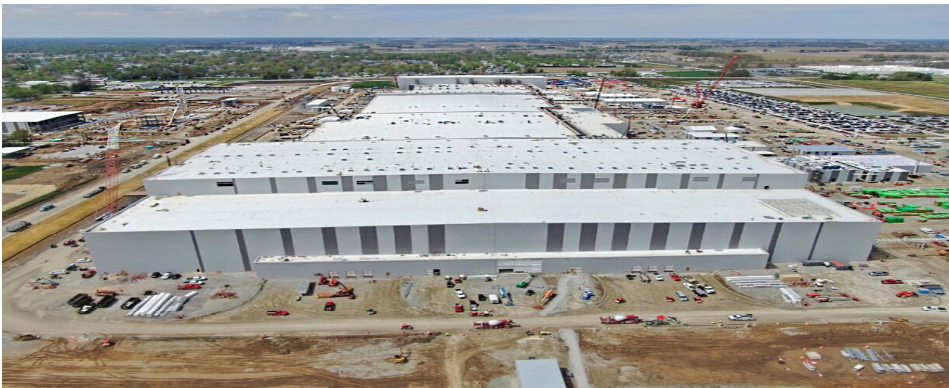
Stellantis / Samsung JV battery manufacturing plant in Indiana - $6.3 billion total investment
