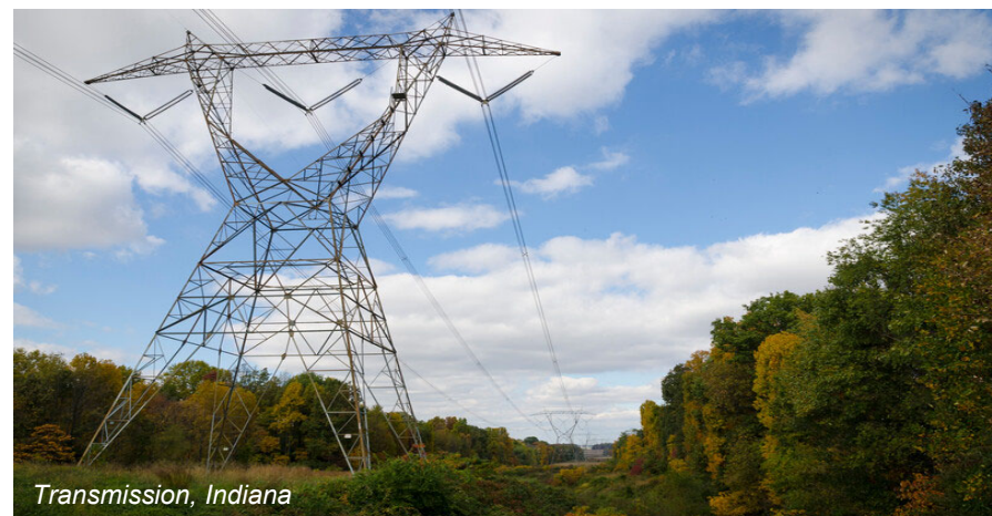
Smith Energy Complex, North Carolina
