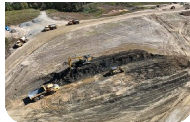
Construction underway at future Person County CC
