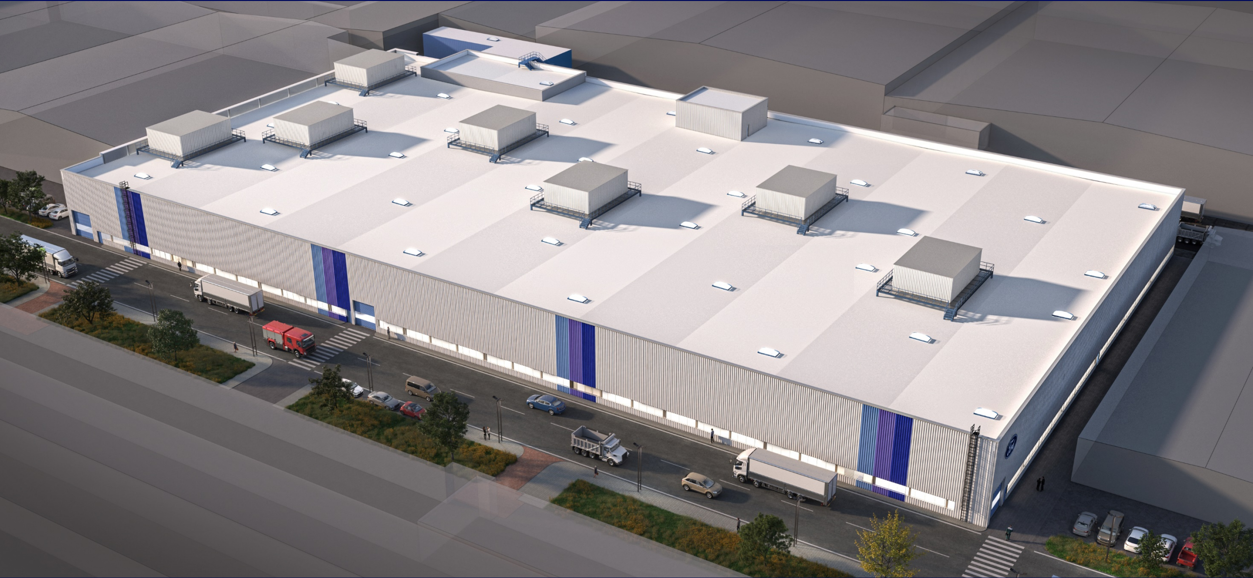
Rendition Of Cologne Electrification Center
