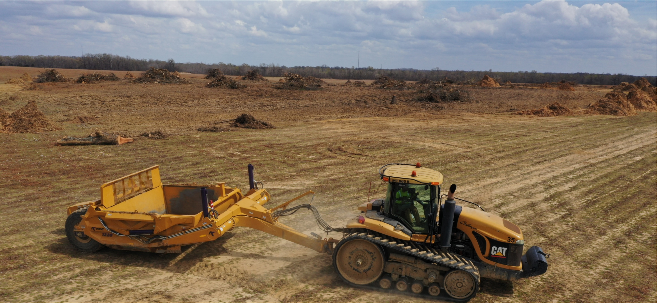
Construction Preparation At BlueOval City
